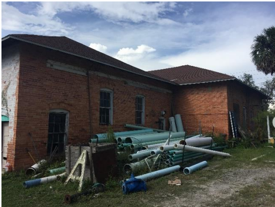
Photo 3: Old Waterworks Building
