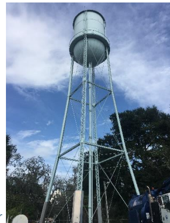
Photo 25: Existing Water Tower
