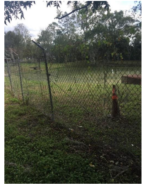
Photo 12: Existing Stormwater Pond
